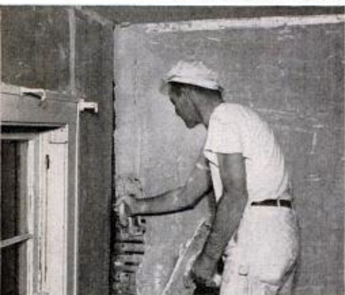
Break in wall is repaired same as ceiling, leveling with float. Roughened surface on plaster formed by float or darby is needed for finish-coat adhesion
